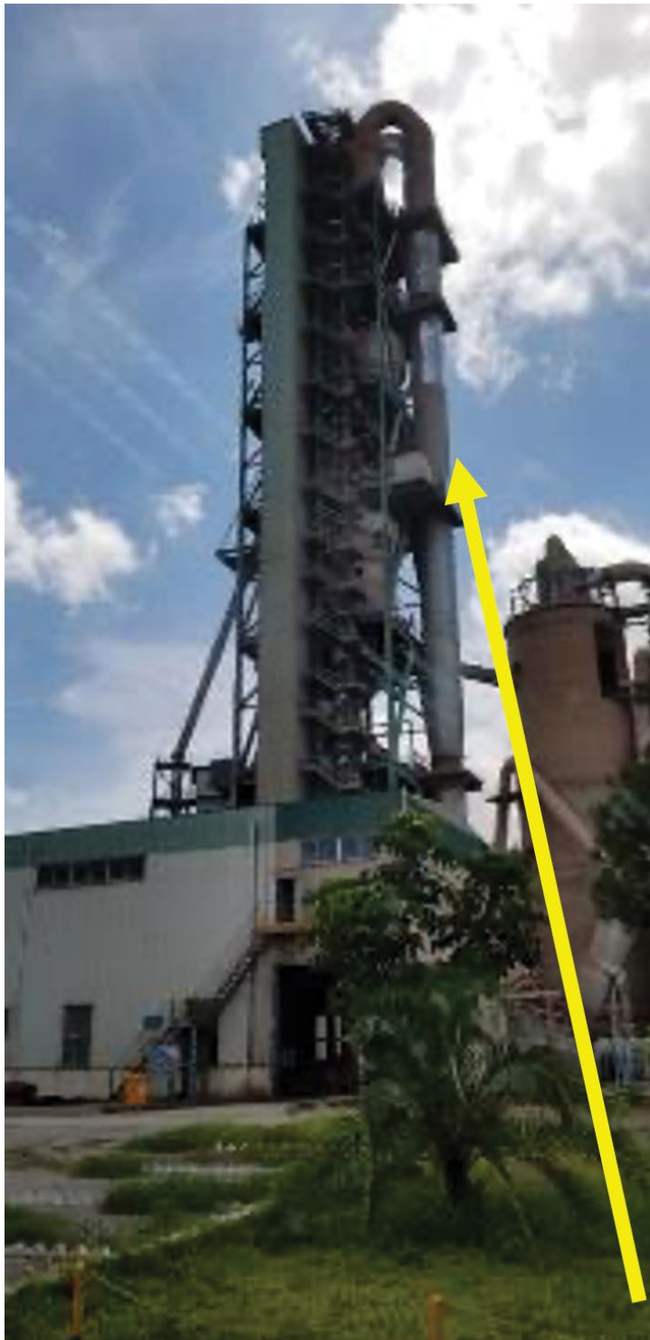
Loading platforms for waste container
